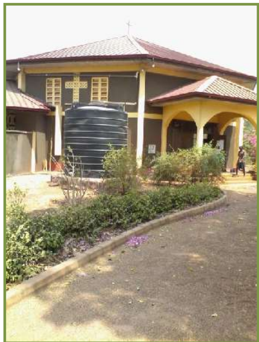
The rainwater cistern
